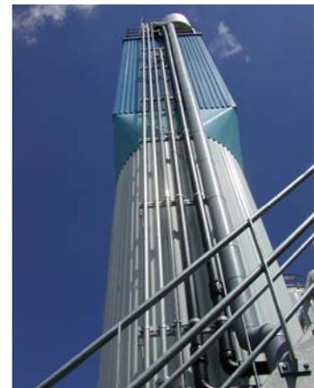
*The full-scale anammox reactor in Rotterdam (NL) converting over 500 kg-N/day.*
